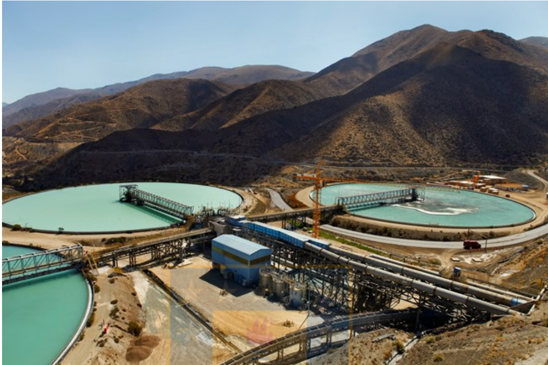
Figure 2: Thickeners in Pelambres mine, Chile. The rightmost thickener shows a short-circuit in gray color at center of the unit. Reprinted from CENTRA Ingeniería Adquisiciones Construcción, by CENTRA Ingeniería Adquisiciones Construcción, Retrieved October 20, 2018, from http://www.centra.cl/construction-en/mining3-en/ . Shows with permission.
