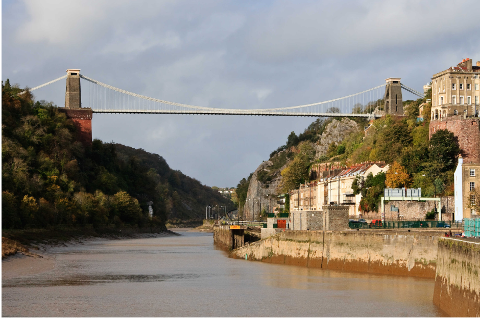
Fig. 1: The Clifton Suspension Bridge in Bristol, UK. https://en.wikipedia.org/wiki/Clifton_Suspension_Bridge
